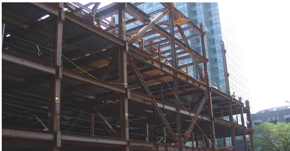
Structural stub-outs on the west side of the structure await the construction of phase 2 of the podium.
