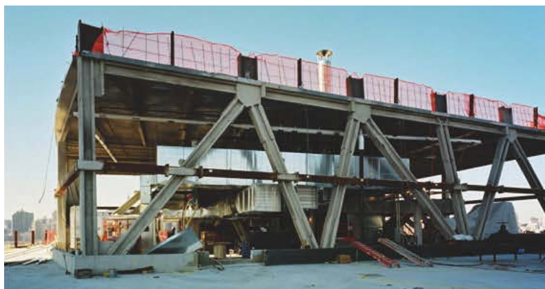
Below: Transfer trusses transition the columns from the future office tower to the columns of the podium structure.
