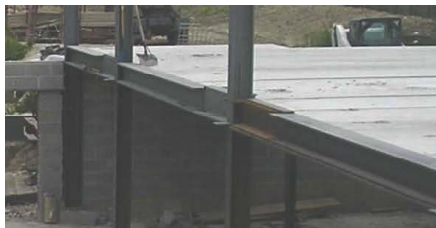
Figure 1. Wide notches in the beam flanges allow the plank to be dropped in and slid into place.
